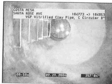
Photo: 30b, Tape/Media No.: 002, 00:00:00 257.33FT, Manhole
